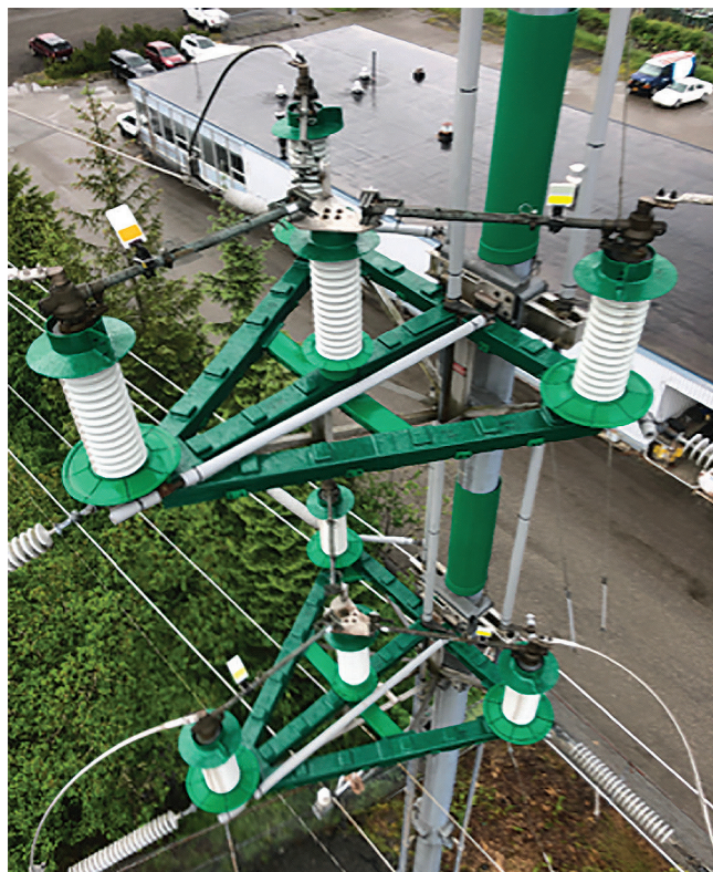
69-kV vertical switch after the application of new avian protection. The green color is part of the design that provides ultraviolet protection for a 25-year life for the polymer pieces.
