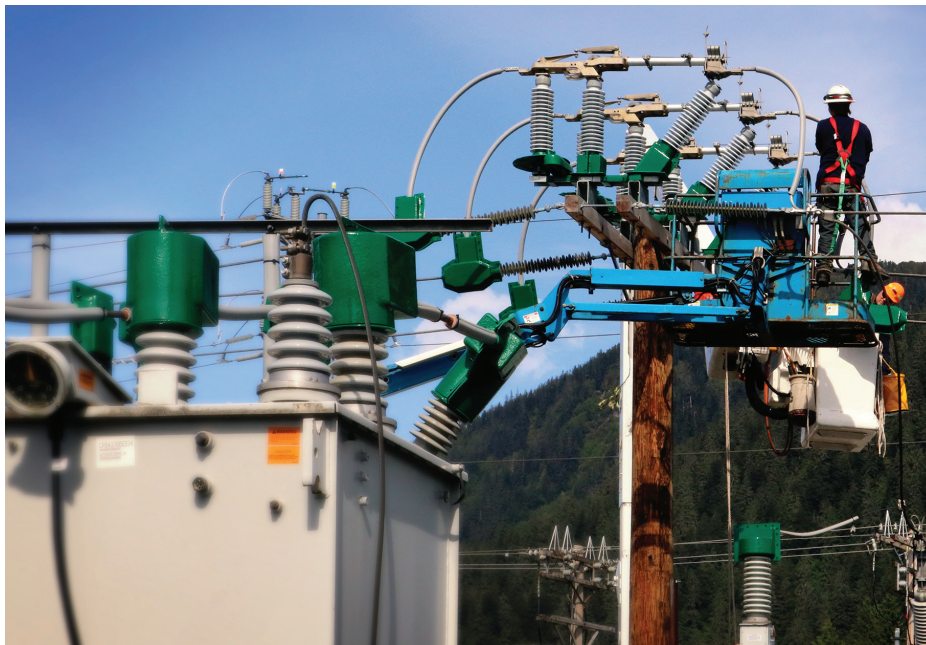
AEL&P line crew inspecting and admiring their installation of the new wildlife protection products.
